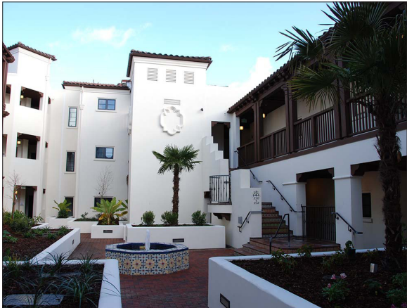
Landscaping on garage top with tall planters is not desirable
