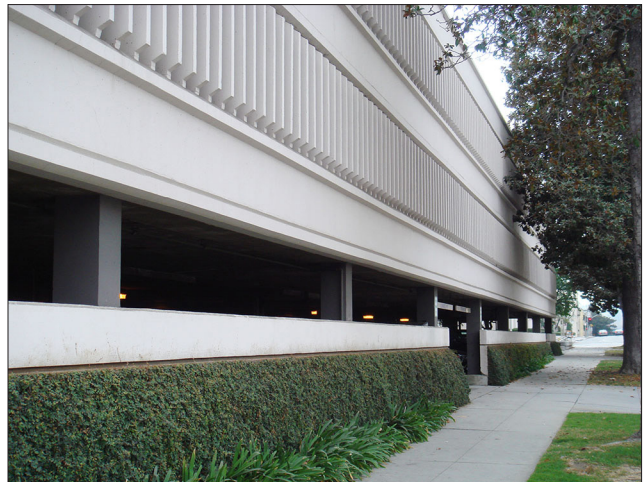
Cast-in-place concrete incorporating precast concrete elements
