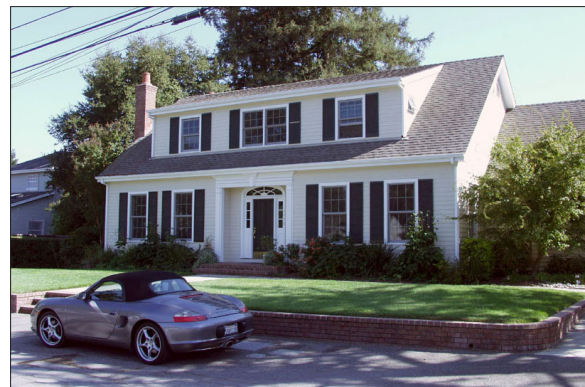
Same house after second floor addition within the roof form with shed dormer and side windows)
