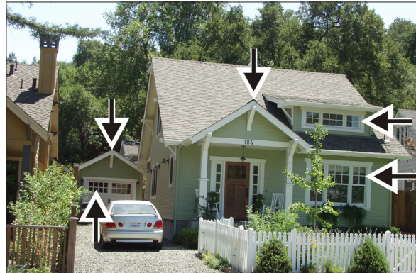
Same house after second floor addition within the roof form with shed dormer and side windows)
