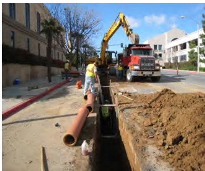
Sewer and water pipe replacement would require excavation and removal of existing pipelines, replacement and/or repair of inadequate pipe segments, and replacement of pavement, sidewalk, and landscaping disturbed during construction.
