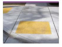
Curb ramps allow for smooth transitions between the sidewalk and street level. Curb ramps are important for those with special mobility needs, strollers, and many other users. Ramps must be built to current ADA standards.
