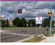
A pedestrian hybrid beacon, also known as a High-Intensity Activated Crosswalk (HAWK), is a signal designed to increase safety for people crossing at unsignalized locations on multi-lane roadways. When the button is pushed, the beacon will flash yellow to alert drivers to prepare to stop. It will then turn solid red to indicate drivers should stop. Once it begins flashing red, drivers may continue once the crosswalk is clear.
