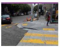
The size of the curb radius (angle of the corner) has an impact on the speed of turning vehicles. A reduced corner radius creates a tighter turning movement and therefore reduces turning speed. Reducing turning speeds to about 15 mph is important as corners are where drivers are most likely to encounter people crossing. Curb extensions/bulb-outs are one way to reduce corner radii.
