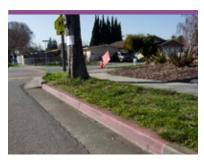
Curb colors indicate parking/ loading restrictions along segments of curbs. In most cases, these are accompanied by signs providing additional detail about the restriction. Existing and proposed changes are noted on improvement plan maps. The length of the curb designation should be determined in accordance with City standards.
