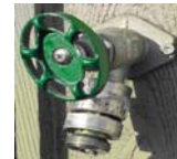
Hose bib with vacuum breaker installed
